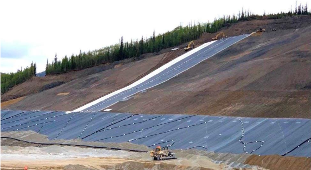
Figure 9: Geomembrane and GCL liner deployment on the steep west slope of the Eagle Gold VLF (reproduced from Smith and Konrad 2025 with permission)
