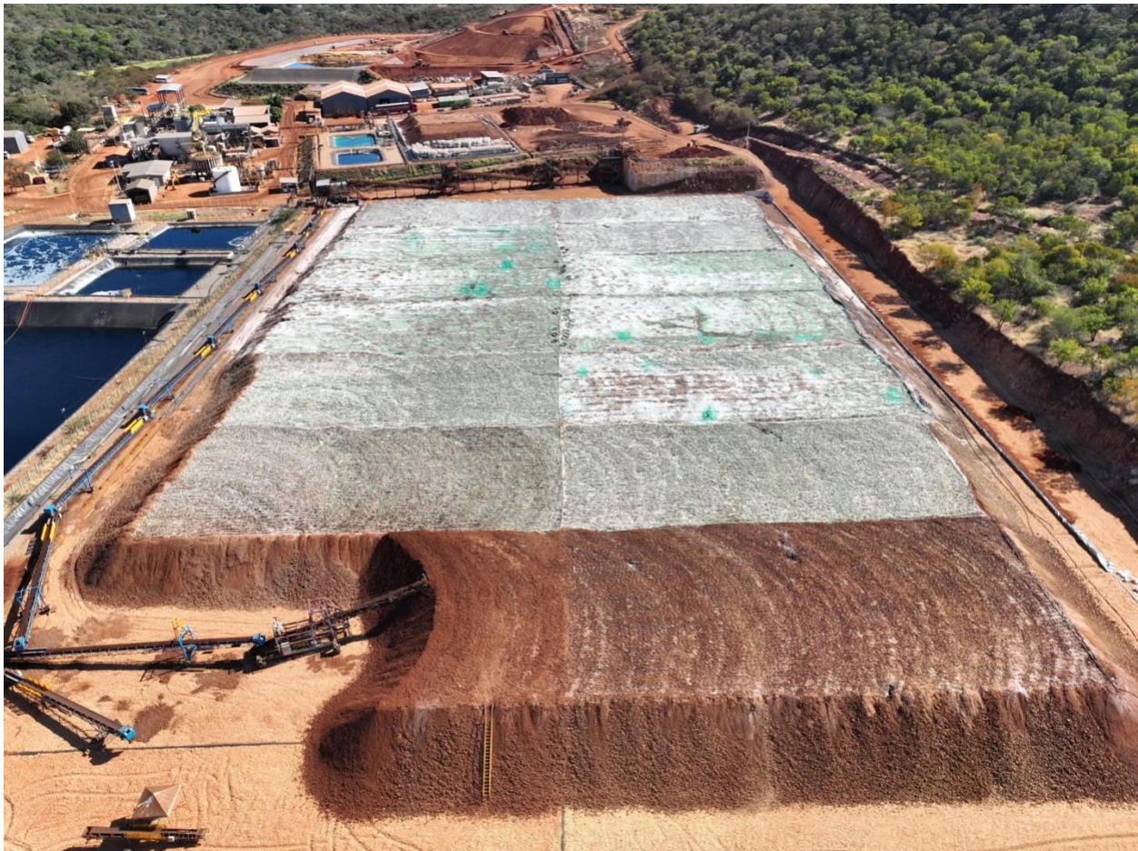
Figure 31: The Piauí dynamic nickel heap leach facility in Brazil (source: Brazilian Nickel Ltd, used with permission)
