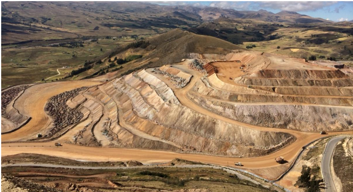
Figure 17: Advance stacking with truck and dozer on a ROM heap
