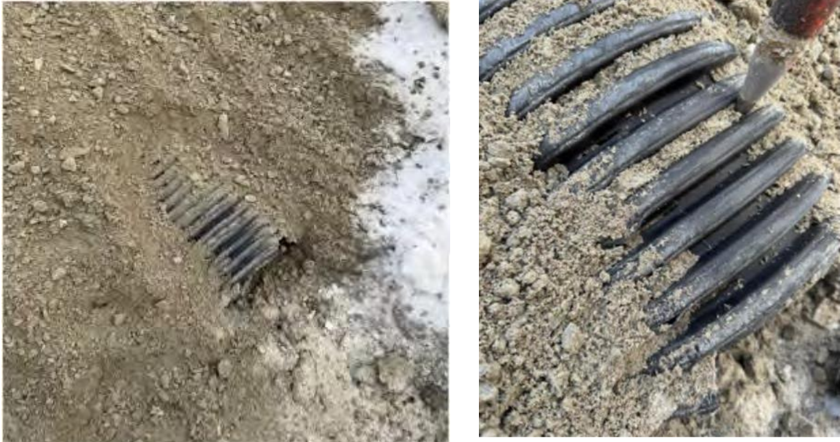
Figure 11: The PLS collection system for the Eagle Gold HLF showing high-sand content drainage material (reproduced from Smith and Konrad 2025 with permission)
