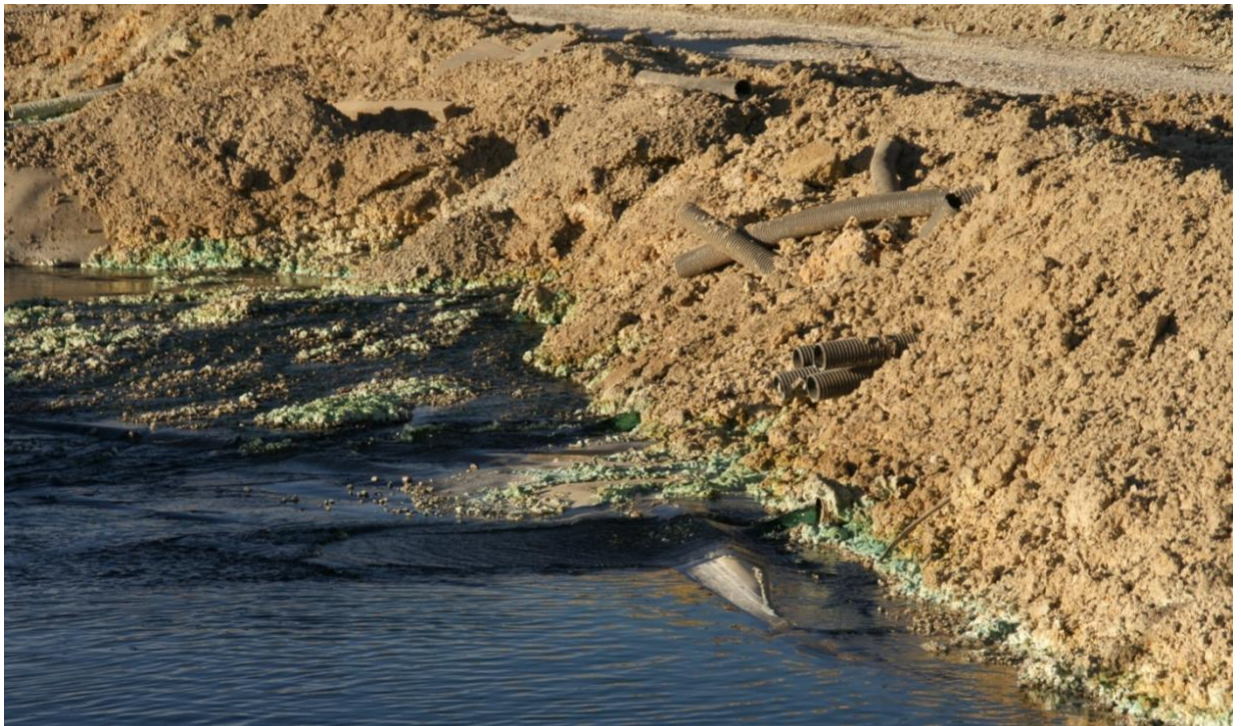
Figure 13: Partial chemical clogging of the overliner at a copper dynamic HLF in Chile
