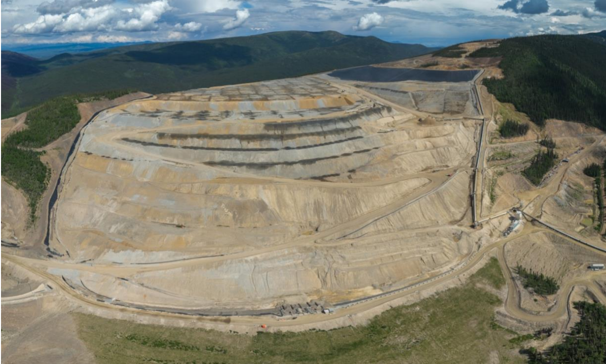
Figure 23: Eagle Gold VLF showing slope irrigation in May 2024. Note the side slope seepage about 100 m vertically below the crest (reproduced from Smith and Konrad 2025 with permission).
