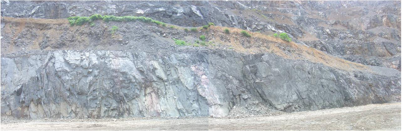
**Figure 18** - Sequeirinho Pit North Wall (shear zone). Note the surface of the shear zone and the consequent effect on the blast results.
