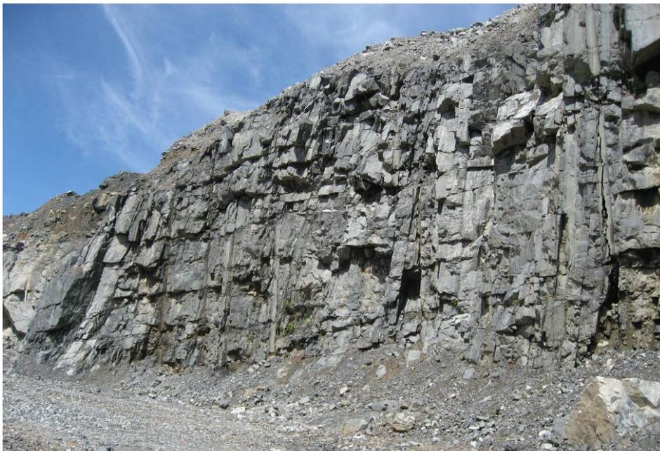
**Figure 19** - Sequeirinho NW Wall in Schist. Note the loose blocks at the crest; half barrels are present along most of the wall.
