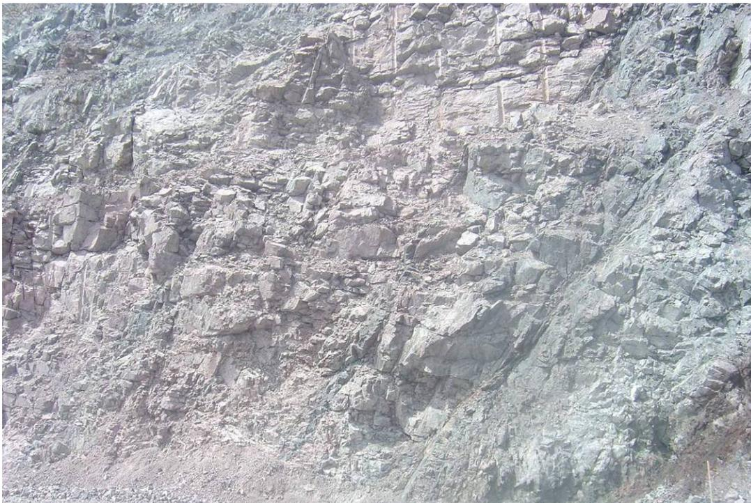
**Figure 17** - Smooth Blasting of a Granite Face in Sequeirinho Pit. Note the Joints intercepting the Half Barrels and forming Rock Blocks.
