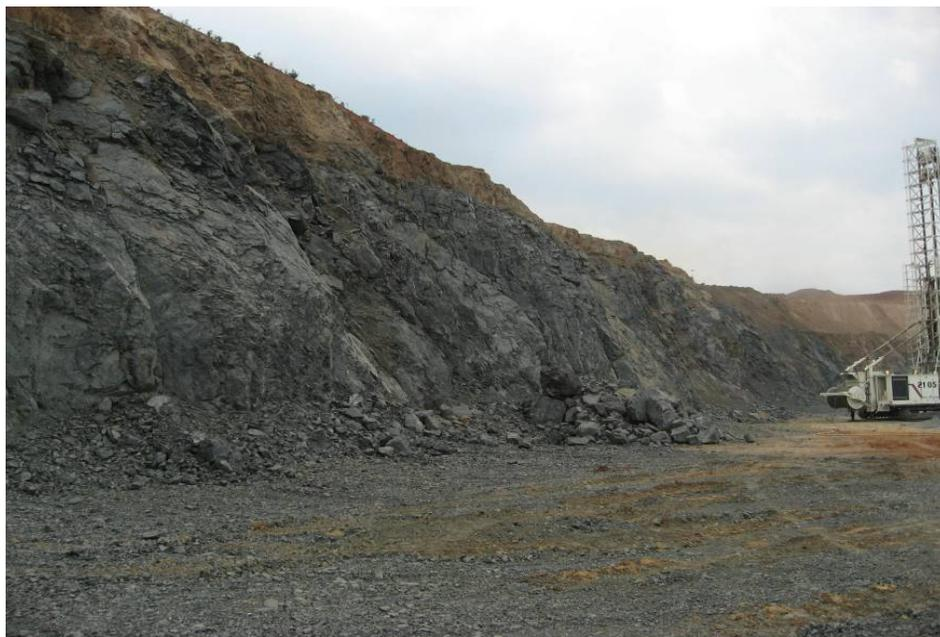
**Figure 12** - Blast Damage in MVAC in North Wall of Sequeirinho Pit
