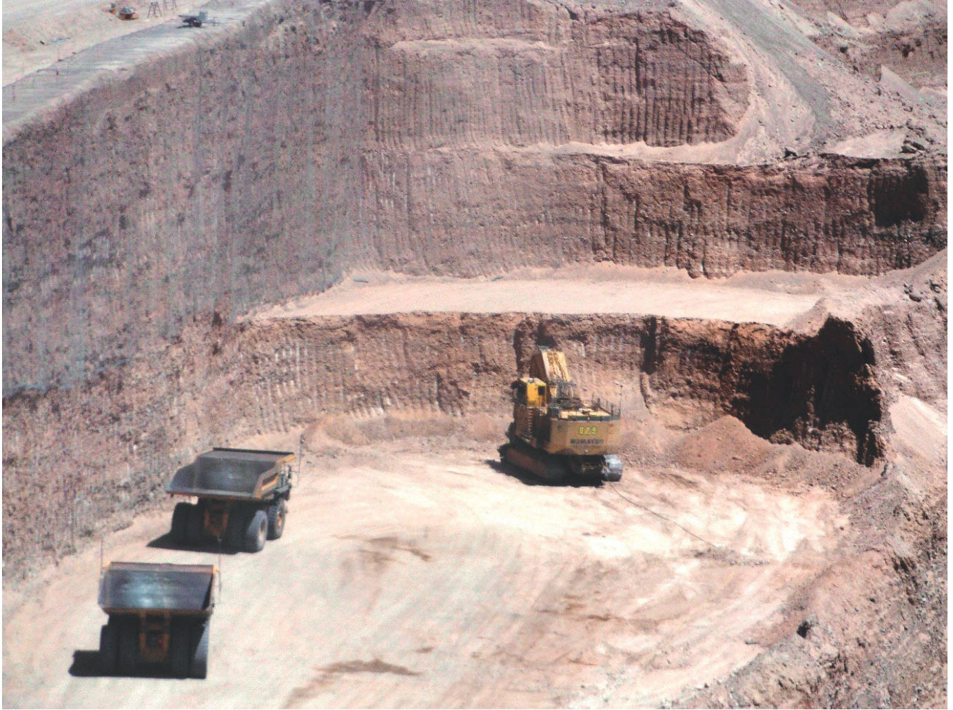
Figure 5: Trial Smart Marker site. 2x marker chains installed behind the vertical double bench on the LHS of the photo (source: Fredes, 2016)
